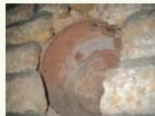
An example of an acoustic jar situated in St Andrew's Church, Lyddington
